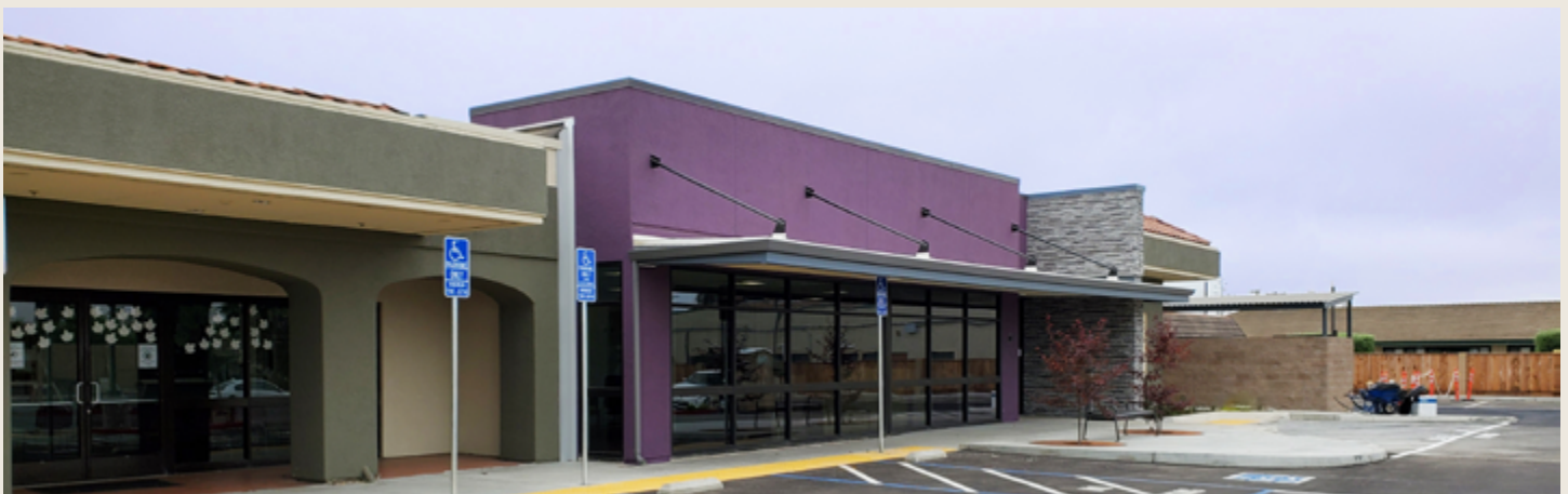
Greenfield Clinic - After
